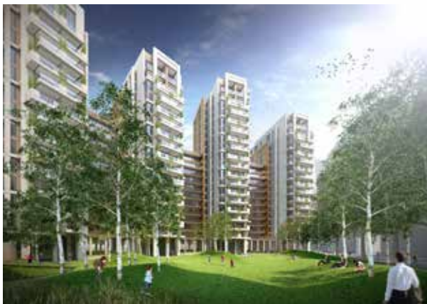
North Wharf Gardens project located in Paddington in central London.
